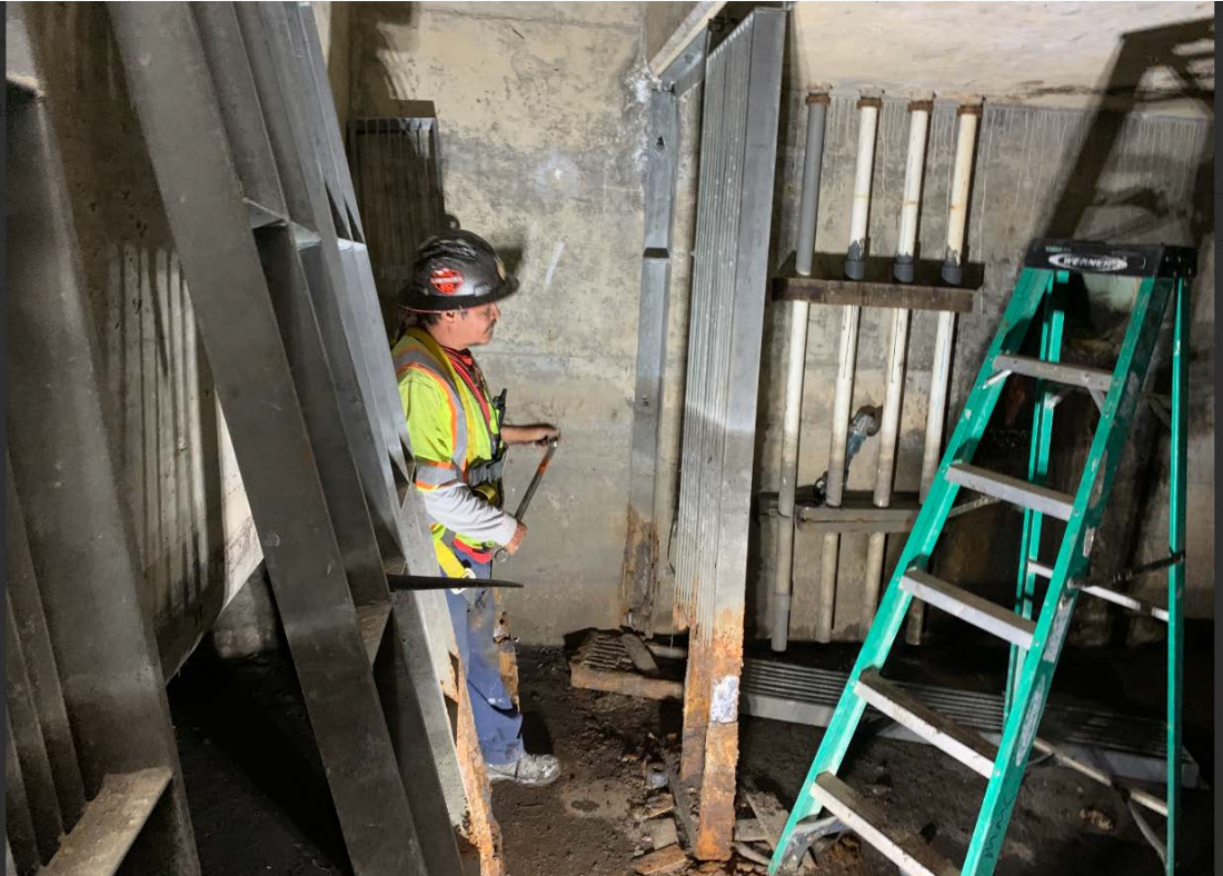
Existing Trash Rack Removals
